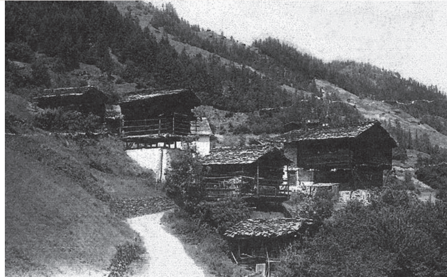
House of the Bourgeoisie of Frasses, right, old chapel, left, in the 1960s
