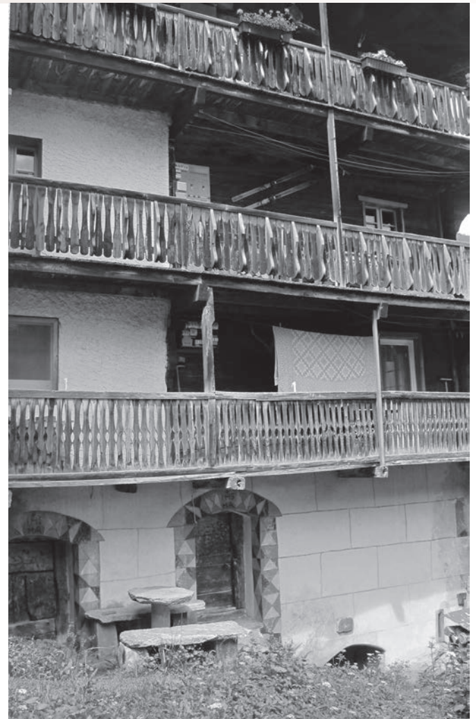
Façade with painted decorations, today
