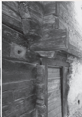
Beams finished with an axe
