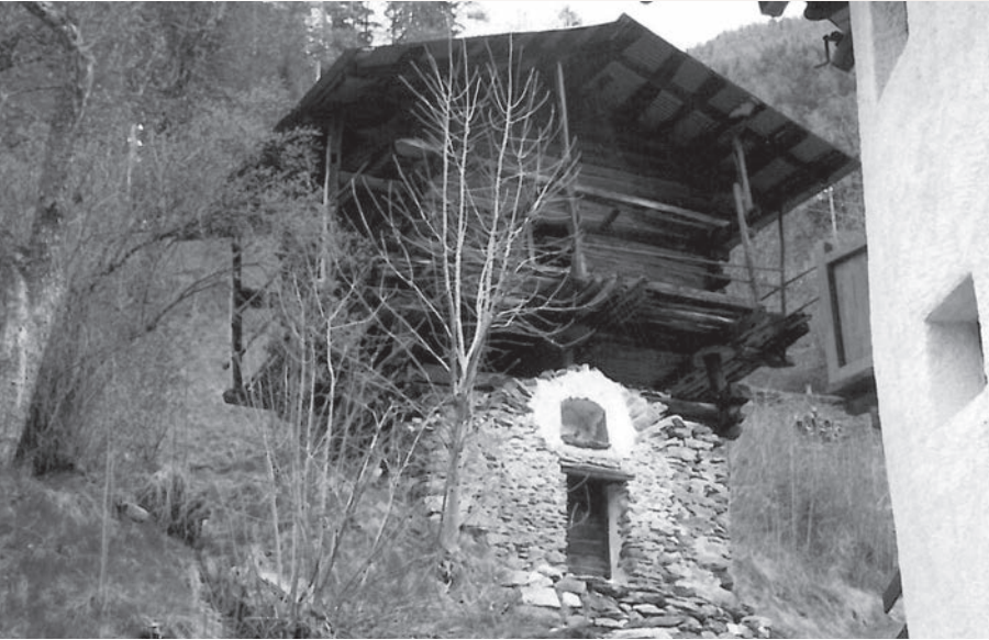
Raccard, before restoration
