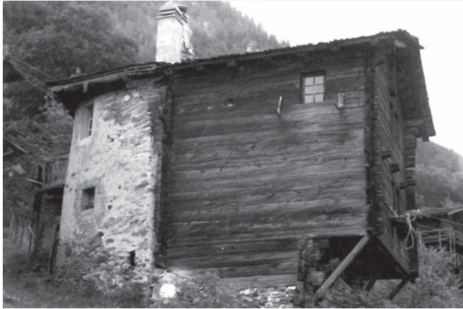
House, before work in 1998
