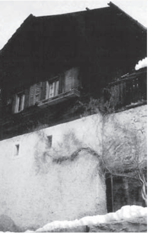
Former Villagers House
