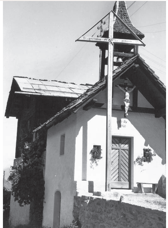
Villagers House and Chapel, in the past
