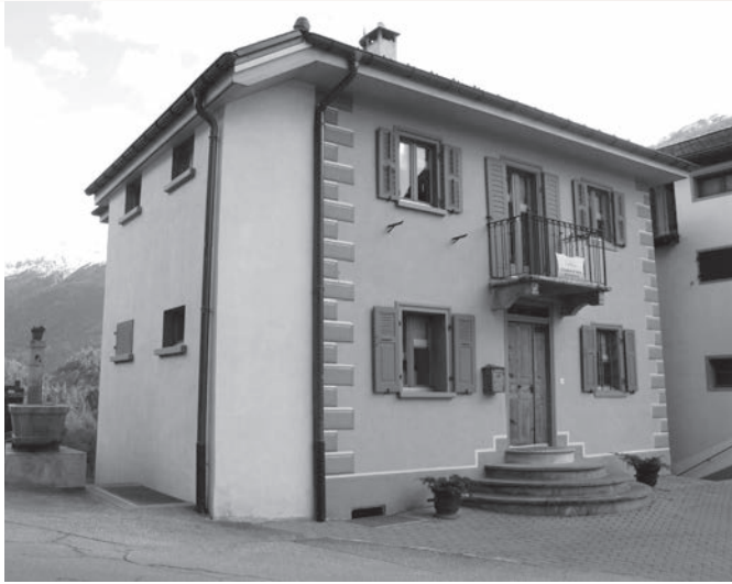
Former Mining house and post office today
