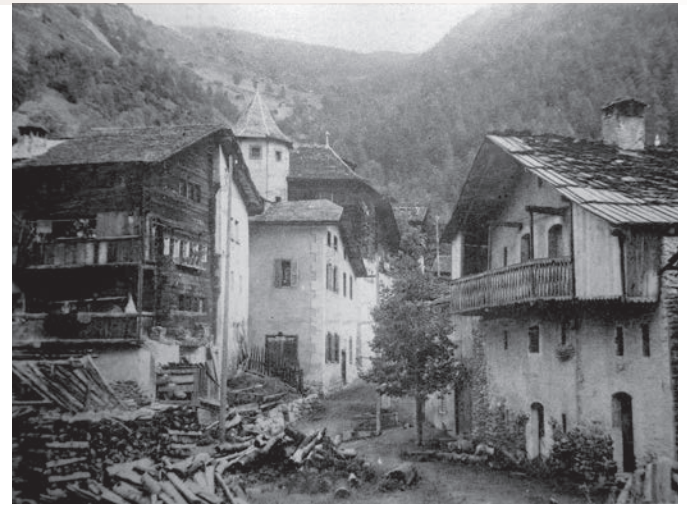
The Gillet House, with its tower left, early twentieth century
