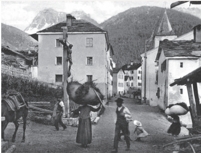
Heart of the village, as it looked rebuilt after the fire
