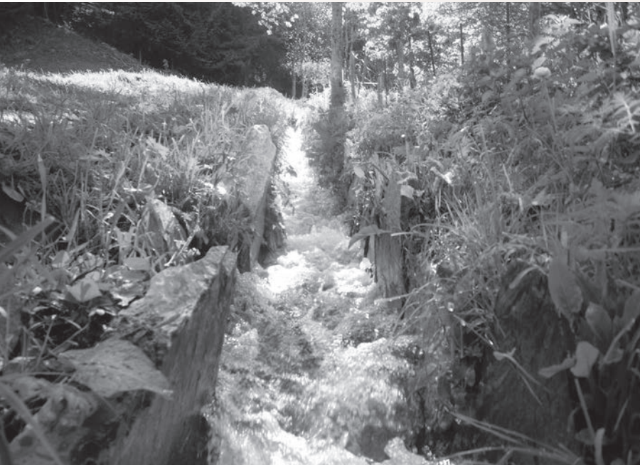
Stonework of the Grand Bisse between Saint-Jean and Mayoux, in summer
