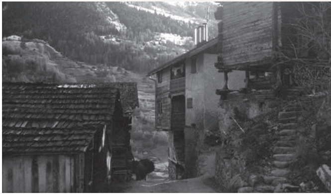
Last farm buildings at Saint-Jean d'en haut, in 1986
