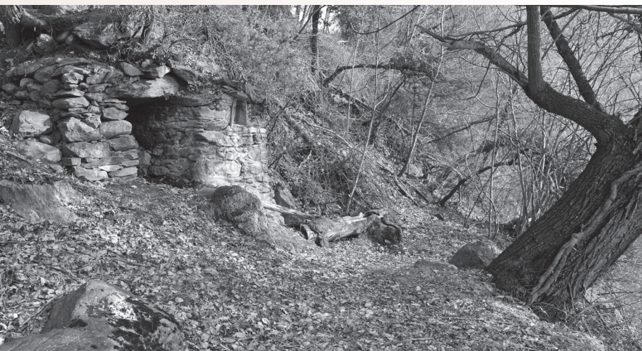
Exit point of the spring water today
