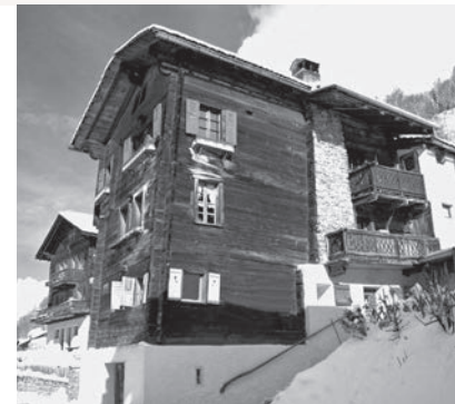
The oldest house today
